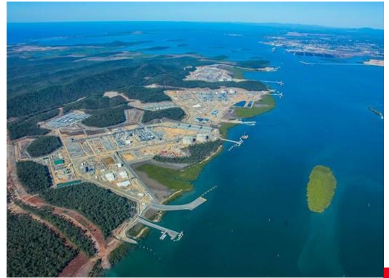
Curtis Island Projects ©Bechtel
